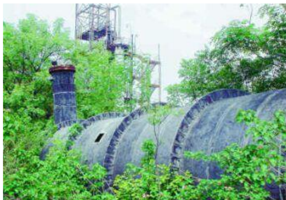
Fig.1.7: The methyl isocyanide tank at Union Carbide Corporation's factory in Bhopal, which leaked in December 1984 causing a major disaster. Waste material dumped in and around the factory is now feared to cause soil and groundwater contamination in the neighborhood of the site.
